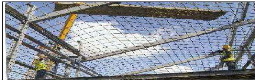
Photographs (above and below) showing application of Net
